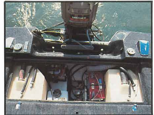
Fuel Tanks & Battery Area with Removable Lid
